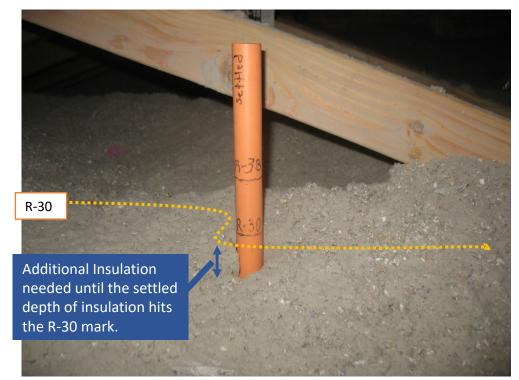
Loose-fill insulation depth and density is verified in at least 6 random locations to show the CF1R value has been met.
