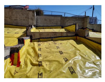
Stego Wrap Vapor Barrier 15 mil Water Vapor Permeance: 0.0086 perms Can be used to stop moisture and radon.
