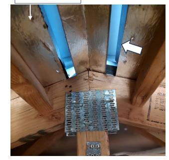
Vented Attic with Traditional Ridge Vent Can use standard ridge vent assemblies. As a 'vaporport' the vent openings could be covered by vapor-open membrane (>20 Perms)
