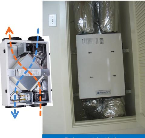
Balanced Ventilation HRV Provides Outside Air (OA) Duct System Manifold 'Home Runs' to the Heat Tous Joist Timber Strand Exchanger and Fan Unit Heat Exchanger and Fan Unit zehr
