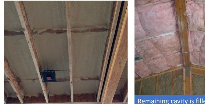
2" Closed Cell Spray Foam is adhered to underside of roof deck.
