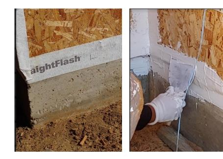
Structural sheathing is ready for a liquid applied membrane, self-adhered membrane, or drainage plane stucco wrap.
