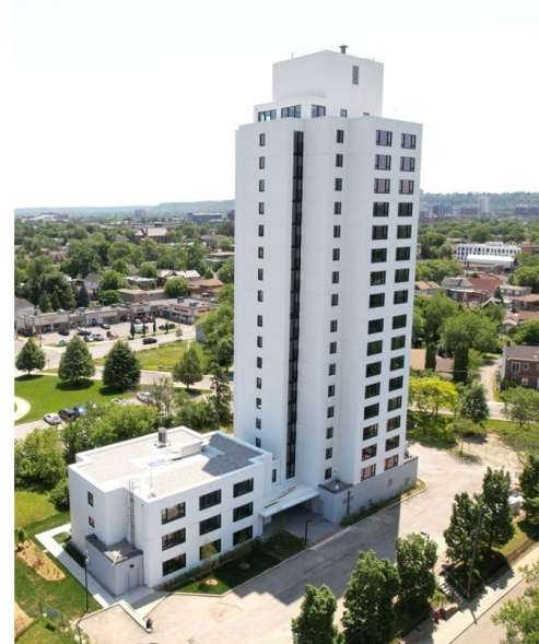
Concrete Frame & Masonry (interior & exterior)
